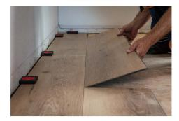
Step 2: Take another long plank, repeat the previous step, insert the long side of plank into long side of previous plank.
