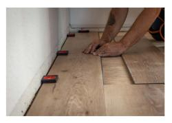
Step 1: Spacers should be placed against walls to maintain proper distance (1/2" - 5/8").
