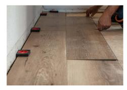
Step 4: Using the drop lock system, drop the short side of the last long plank into the short side of the first laid plank.
