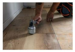
Step 5: Slightly tap on the top of the joint of the short side with your rubber mallet to secure.
